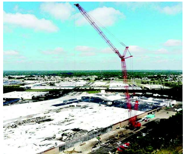
Rebuilding Dayton-Phoenix Group facility.
