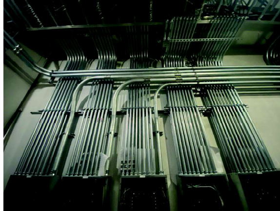
Renovation at the Heraeus Epurio facility in Vandalia.
